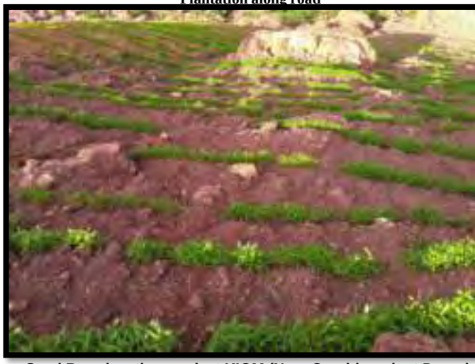
Seed Broadcasting work at KIOM (Near Crushing plant Dump)
