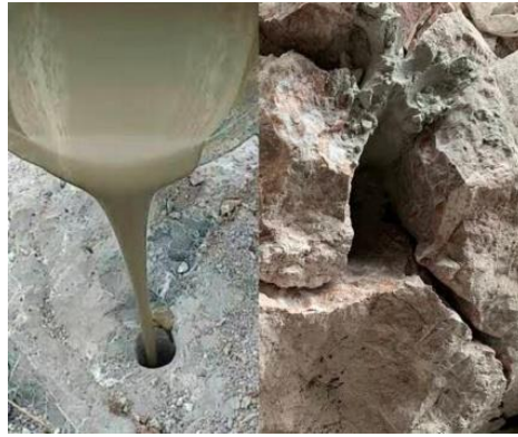
Figure 12: Typical figure showing filling of chemicals for breaking of boulders
