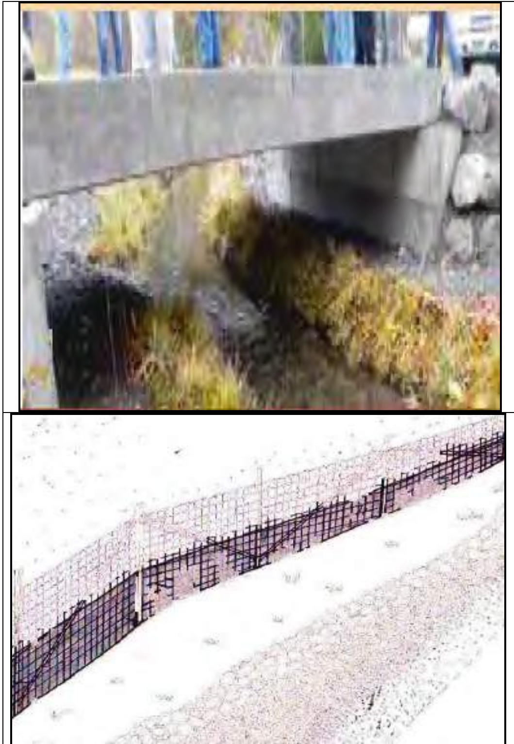
Figure 4.9: Suggestive engineering devices for wildlife management (WII 2016) Top-fish passage; Bottom-fencing along roadside near eco-sensitive zone or National Park
