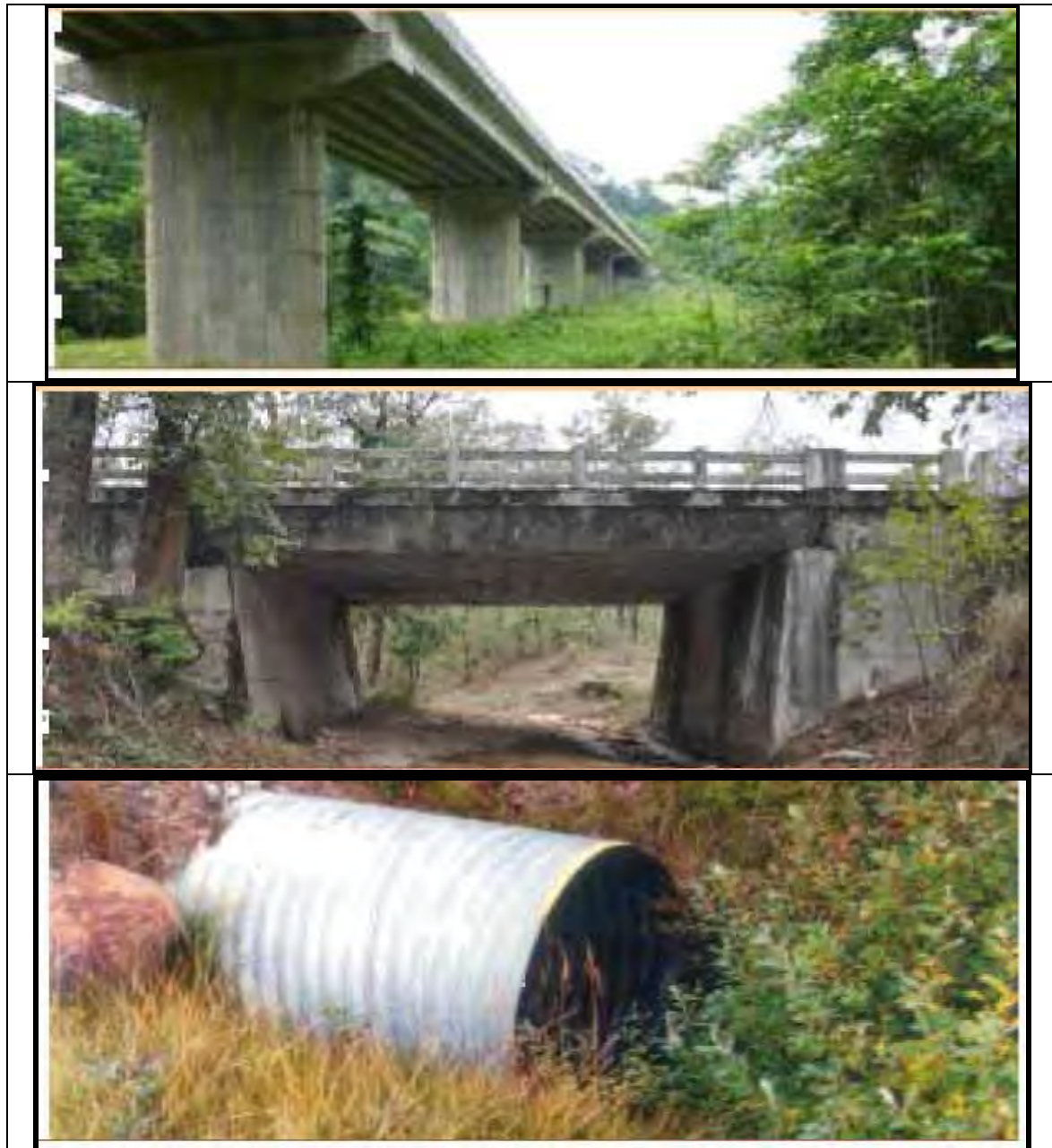
Figure 4.8: Suggestive engineering devices for wildlife management (WII 2016) Top-underpass, Middle-Box culvert; Lower-Pipe culvert
