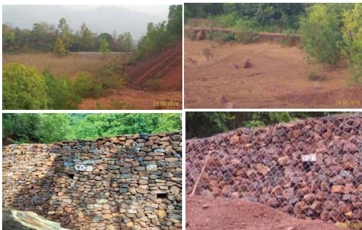
Fig.4.4: Check Dams at Barsua Block
