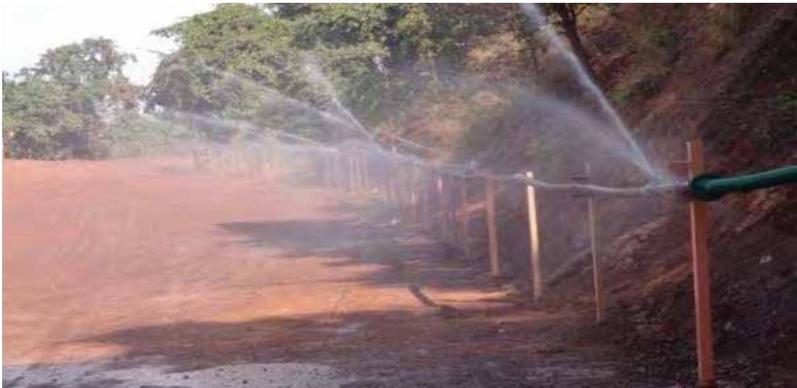
Fig.4.1: Fixed Sprinkler Alongside Road In Kalta Mine
