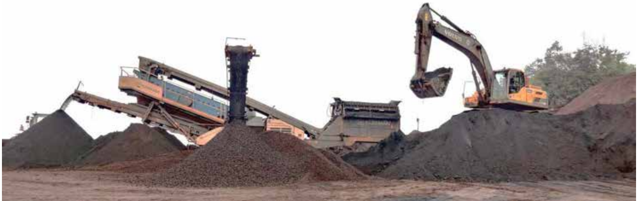
Fig. 2.2: 300 TPH Mobile Screening Plant in Operation at Kalta Mine
