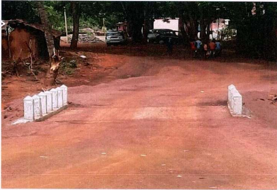
Construction of Culvert to avoid surface water contamination
