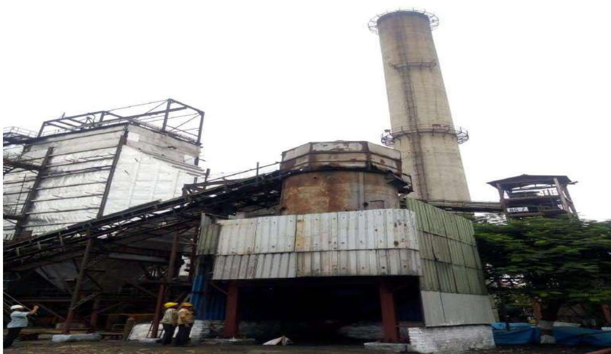
Bagasse Carrier Belt covered by hood to avoid the fugitive dust
