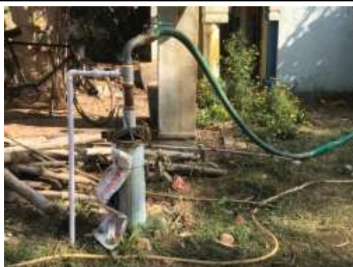
Dom. Bore Well with Submersible Pump 24°24'06.34"N, 81°10'58.14"E
