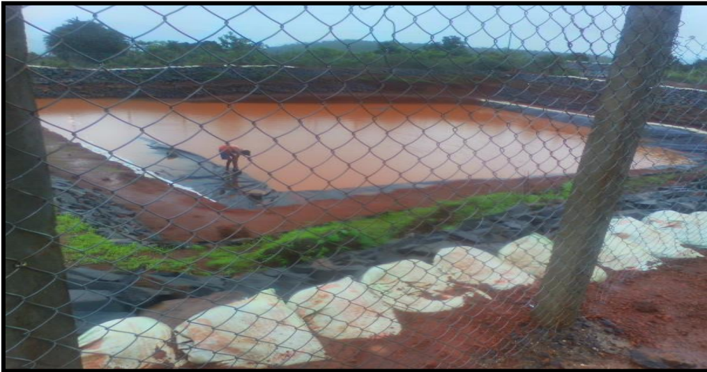
Pond at Nivi: while plastic liningbeingdone
