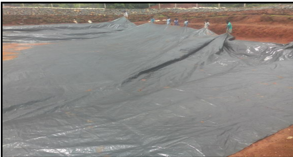
NiviThakurwadi pond lining in progress
