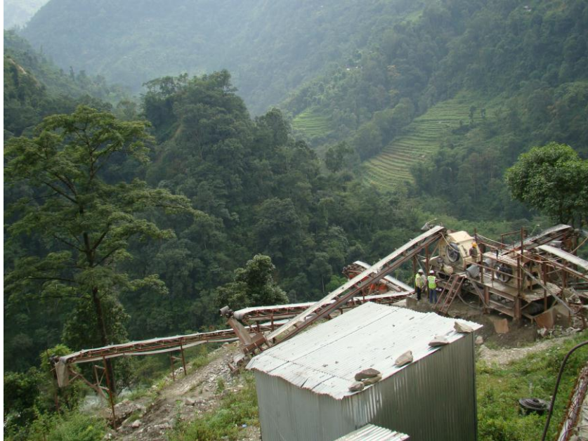
Photograph-1: Stone Crushing Unit near Power House Site
