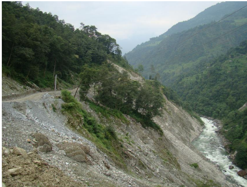
Photograph-2: A view of approach road to barrage/adit site
