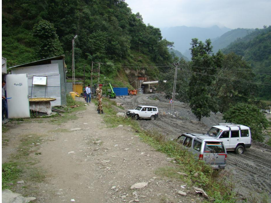
Photograph-3: A view of Adit
