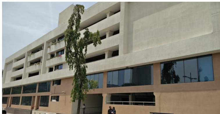
Figure 2-6: Photographs of Building-5 (T1-P01) - Constructed and Operational
