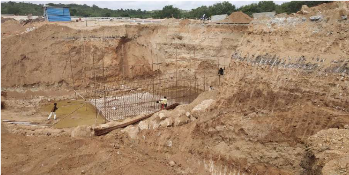
Fig: Construction of Elephant Corridor on Bengaluru-Tirupati Highway (NH-206)
