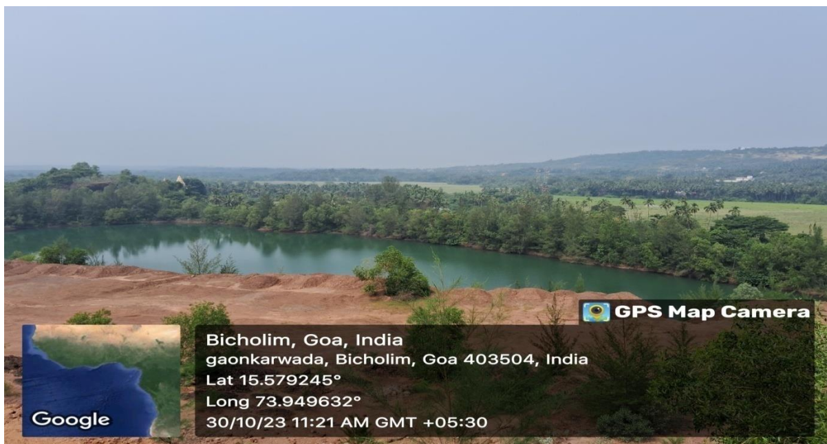
Figure 4: Rainwater stagnant in the mined out pit
