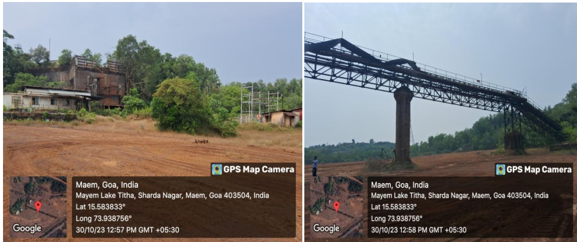
Figure 8: Crushing and Screening Units
