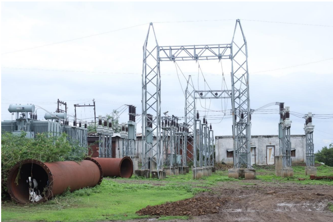
Electrical 33 KV Switchyard of stage-I at Rigaon Tal: - Muktainagar, Dist.:- Jalgaon
