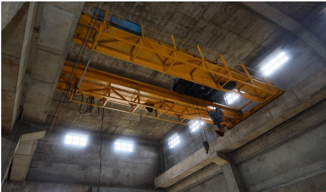
EOT arrangement at Pump House of stage-III at Islampur Tal: - Jalgaon (Jamod), Dist.:- Buldhana
