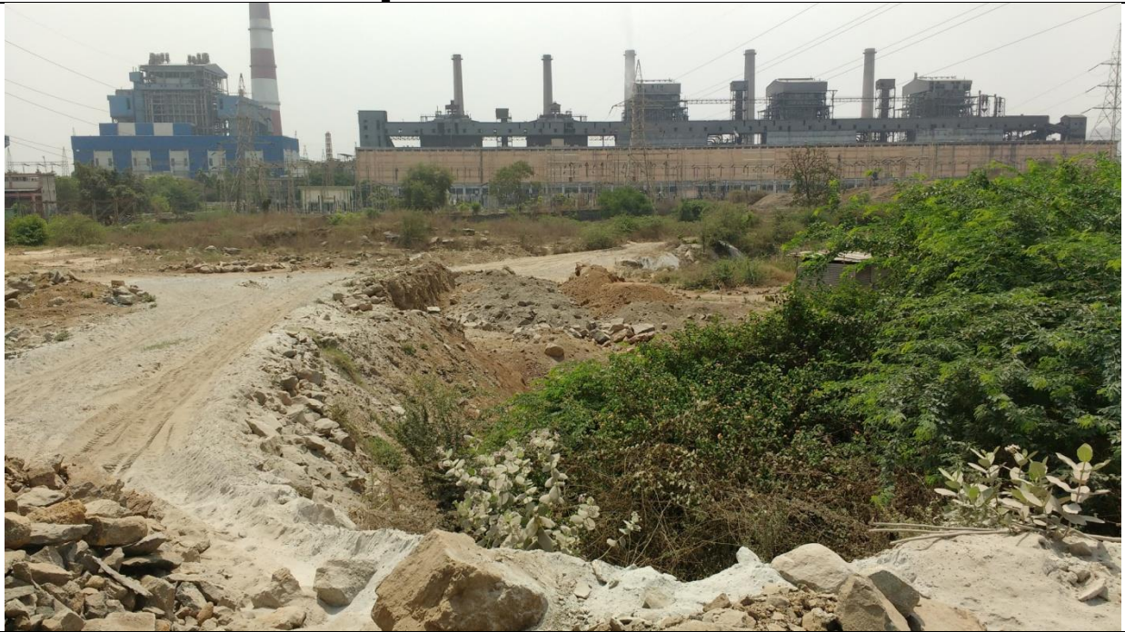
8. Loose ash material on the sides of bund
