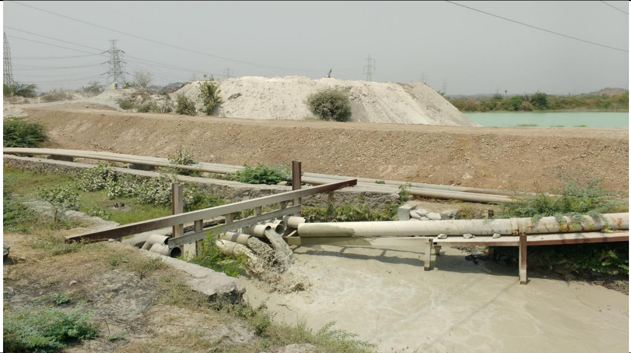
9. Lean slurry discharge
