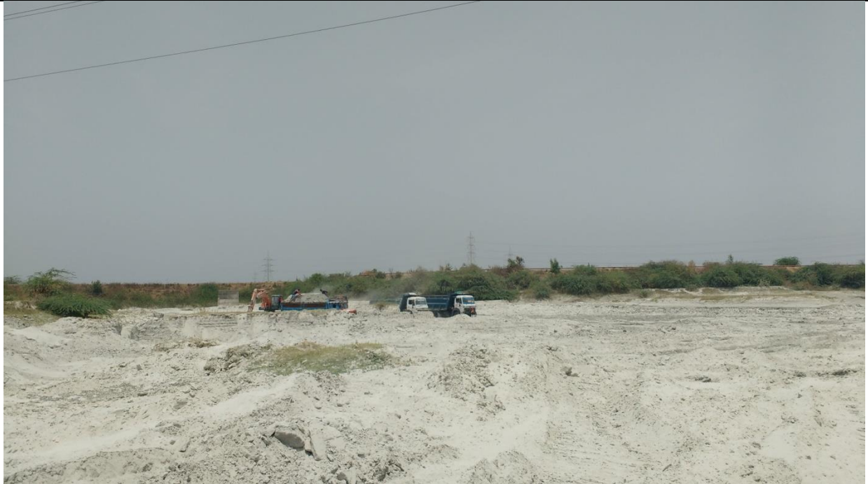
12.Dry ash loading into trucks
