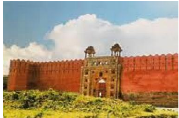
Figure 4. Nagardhan Fort , Ramtek
