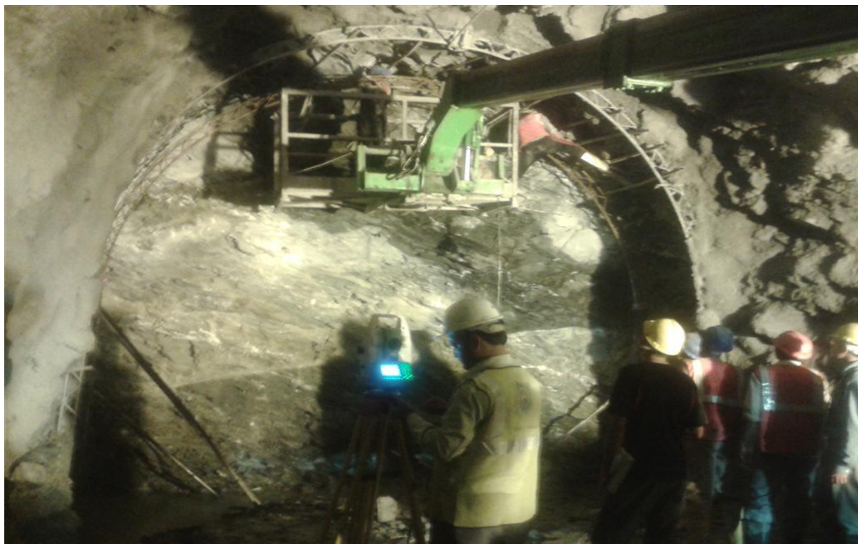
View of Face-4: Lattice Girder erection is under progress
