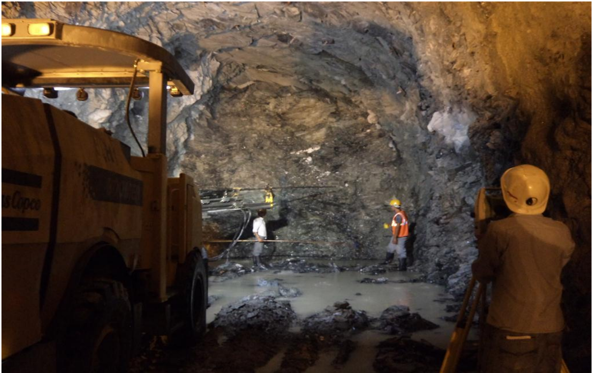
Face Drilling and Profile marking at HRT-Face-3 is under progress
