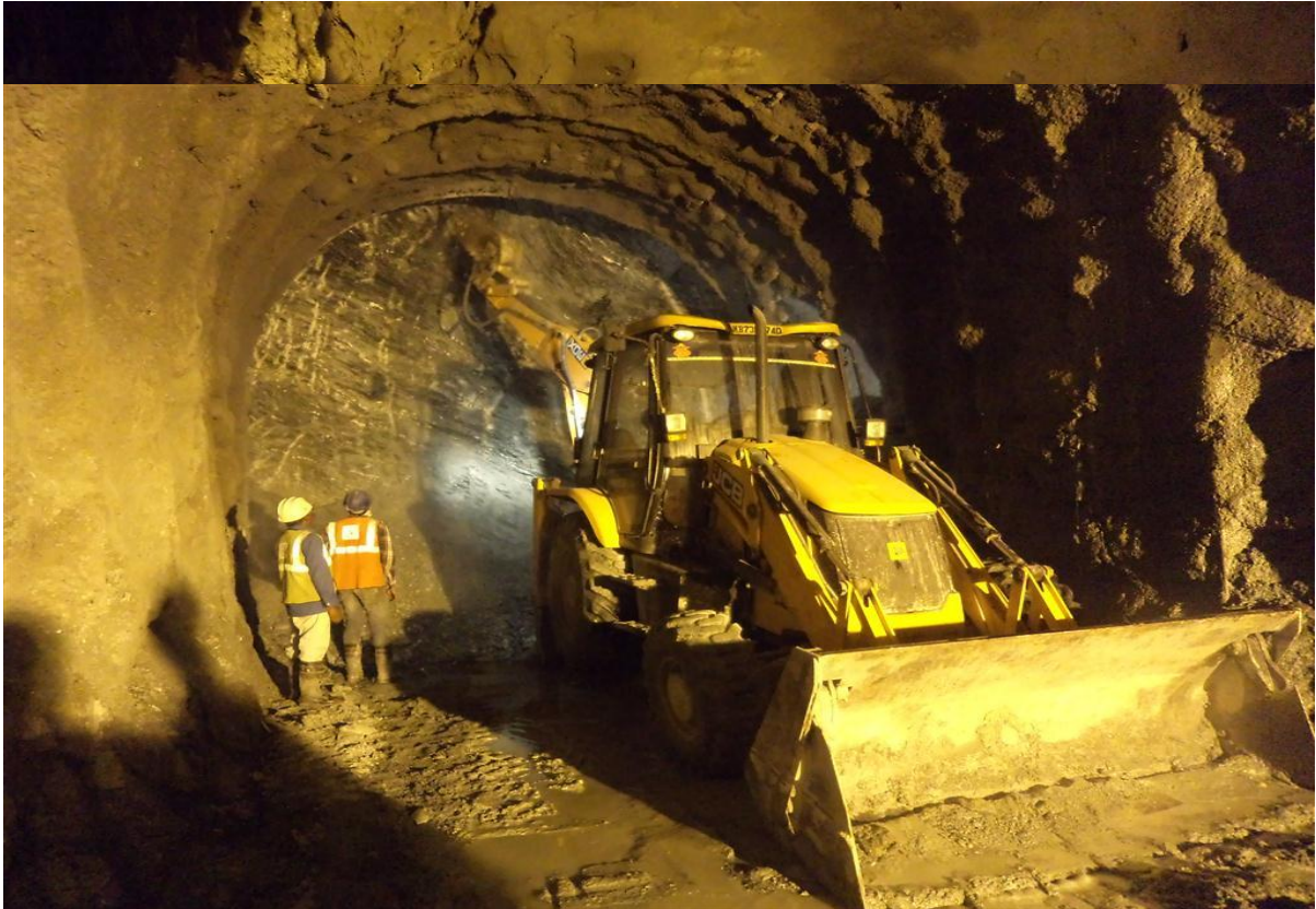
Drilling Works at HRT-Face-1 is under progress HRT-Face-2 Scaling work under progress
