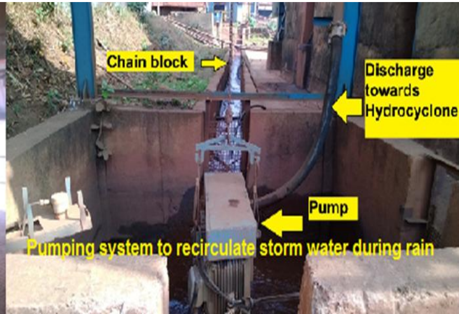
Tailing Dewatering Plant and Water Recirculation Arrangement
