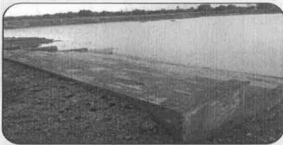
20 Trips of stone was provided for this Construction work
