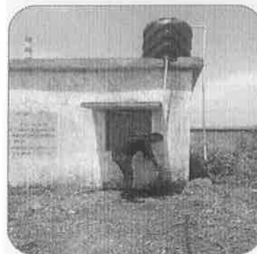
Drinking water pipeline connection in Primary School.
