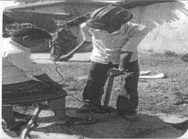
Construction of stairs in Chandan pond at village Kekrabhat.
