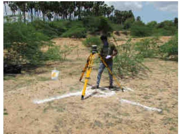
Fig.3. 2 DGPS survey for Ground control Points (GCP) and Drone for Aerial surveying
